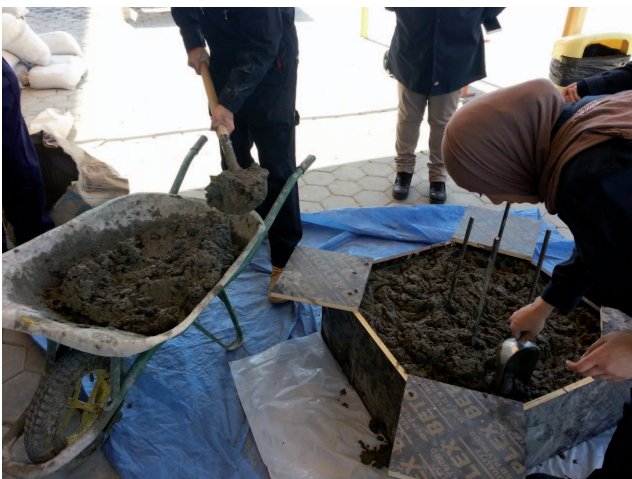
Fig. 2. Students casting concrete for footings
